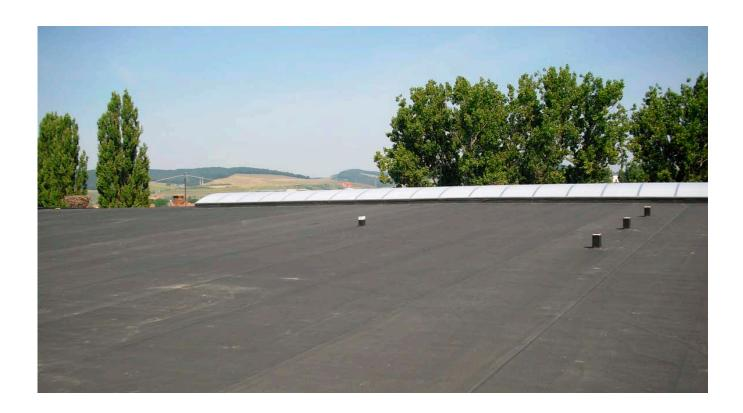
The new ice stadium for the sport park in Marosvasarhely / Targu Mures was built during 2009 with Prelasti membrane as roofing. The roofer that made the installation was the company EBE & CO S.R.L. The total roof area is 4370 m² and this was covered by 8 panels of Prelasti that had been prefabricated in a factory to a panel size of approx 550 m² each.
