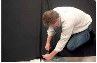
The hot wedge doesn't close the splice where it has started. Therefore the splice at the starting point shall be torn open until full strength is noted.
