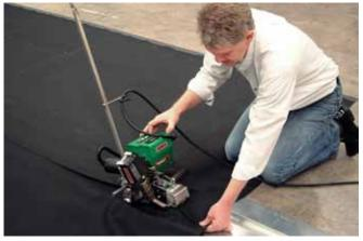
Place the Leister Twinny in position and insert the membrane. Stretch and hold the two layer of membrane when the machine starts.
