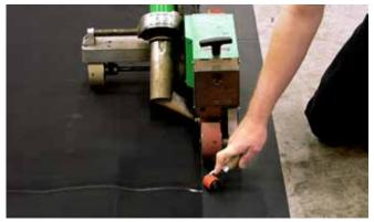
If the Thermobond strip is applied transverse to the membrane lengthway this creates a T-joint. The difference in level must be evened out with Hot melt sealant before bringing on the Thermobond strip as previous described. This areas shall be pressed with pressure roll after the splicing machine passes and re-heats the Hot melt sealant.
