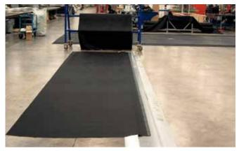
Unroll the first lengthway in required length with the grey Thermobond edge facing upwards, centred in the guiding trench.
