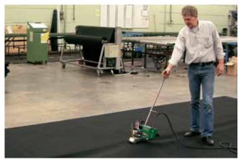
Always control and steer the machine as the splicing goes on. Sometimes the machine needs to be slowed down manually to avoid separation between the membranes.
