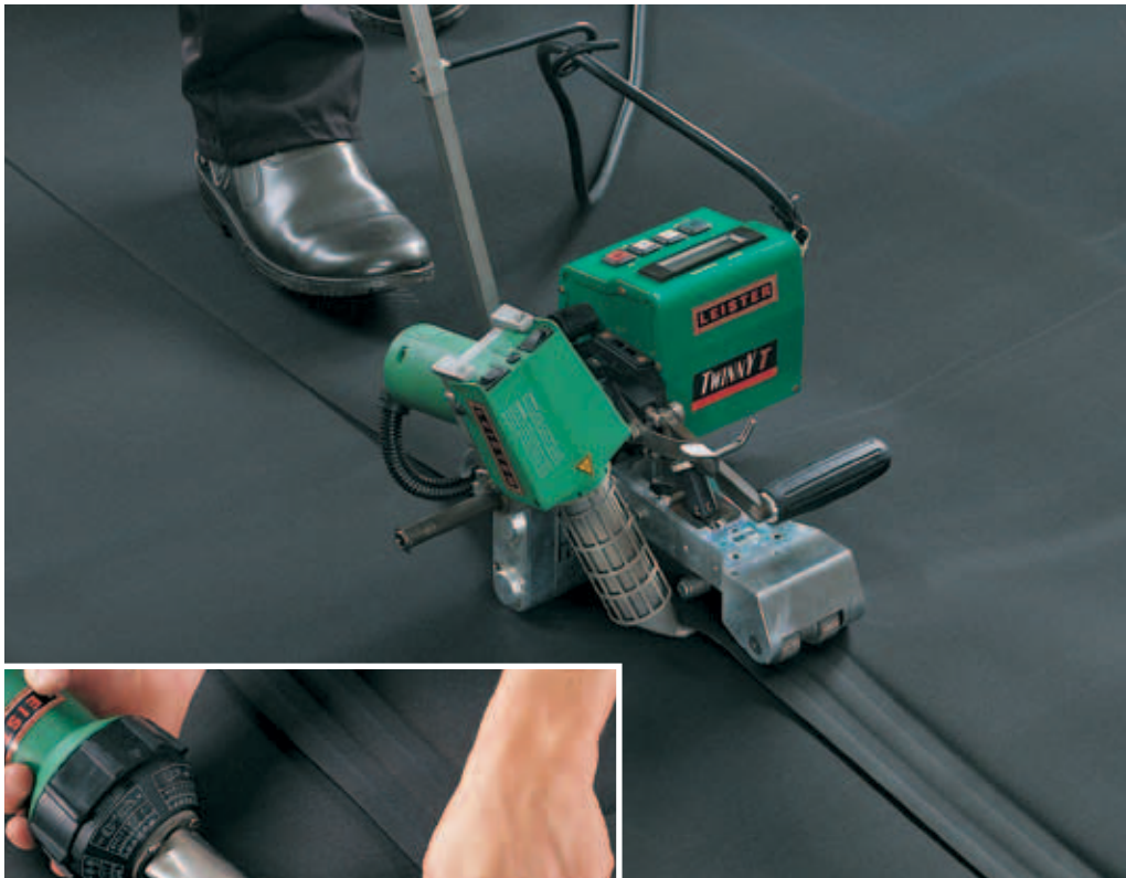
Seams with air pressure test channels are produced with dual hot wedges. The dual wedge provides easy air pressure testing of seams both immediately after installation and after many years of service.
