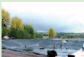
2004 Djupdalen Landfill, Karlstad, Sweden Aeration pond for leachate water. 4.800 m²
