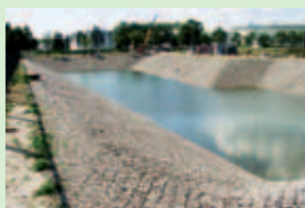
2004 Orlen Co, Plock, Poland Fire fighting pond at petrochemicals storage area. 7.000 m²
