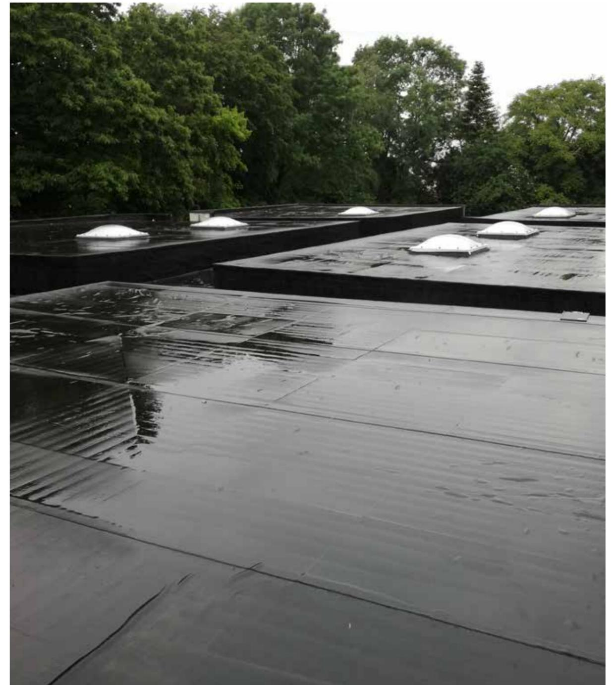
What's unique about RubberShell is its combination of advantages from EPDM based rubber membranes with benefits associated to bitumen felts. This means ease of installation, flexibility and durability, providing waterproofing to any structure. Challenging shapes are no longer a problem to cover quickly and easily with a reliable and visually verifiable result.
