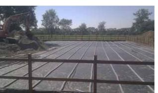
filled with a special sand mixture. In the summer or in dry conditions, water is pumped through the drainage pipes to humidify the equestrian centre. In wet conditions, the system allows the excess water to drain through the pipes. Throughout the year, the substrate has a constant quality thanks to the combination of the drainage system and ElastoSeal waterproofing membranes.
